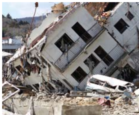
Rubble, trash and puddles of stagnant water abound in crisis-hit Ishinomaki.
